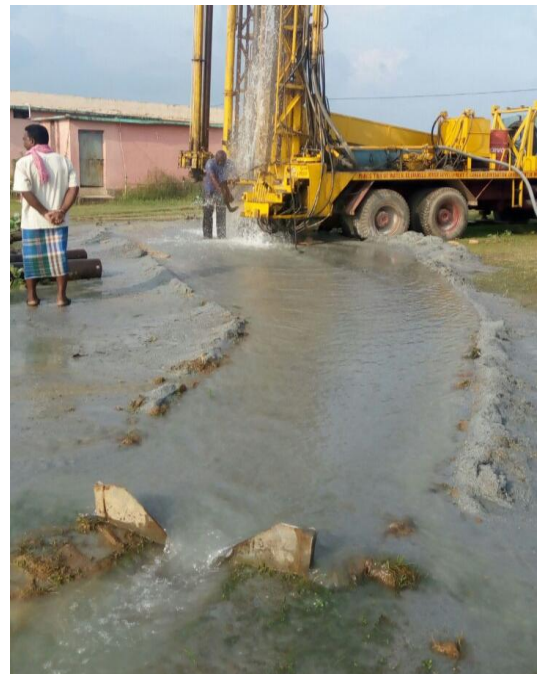
Fig 3.5-Exploratory Well drilled at Nawagaon, Block-Bagbahera, District- Mahasamund (CG), Discharge with 18 lps
