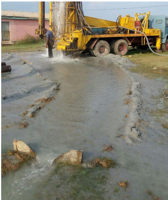
Fig 3.5-Exploratory Well drilled at Nawagaon, Block-Bagbahera, District- Mahasamund (CG), Discharge with 18 lps
